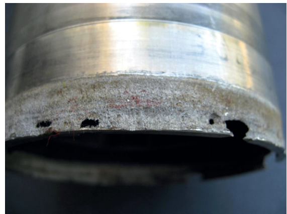
Figure 19 Crevice corrosion of Type 316L stainless steel pump shaft sleeve in natural seawater.
