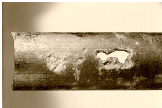
Figure 5 Massive 'black water' corrosion of pipe work under wet lay up because of SRB activity.
