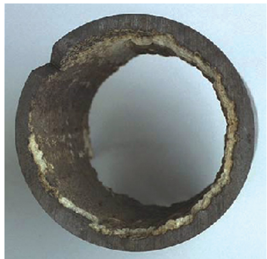
Figure 4 Carbonate scale: dense generally protective scale on a steel water pipe with some corrosion evident as general thinning: Photo courtesy of the author.
